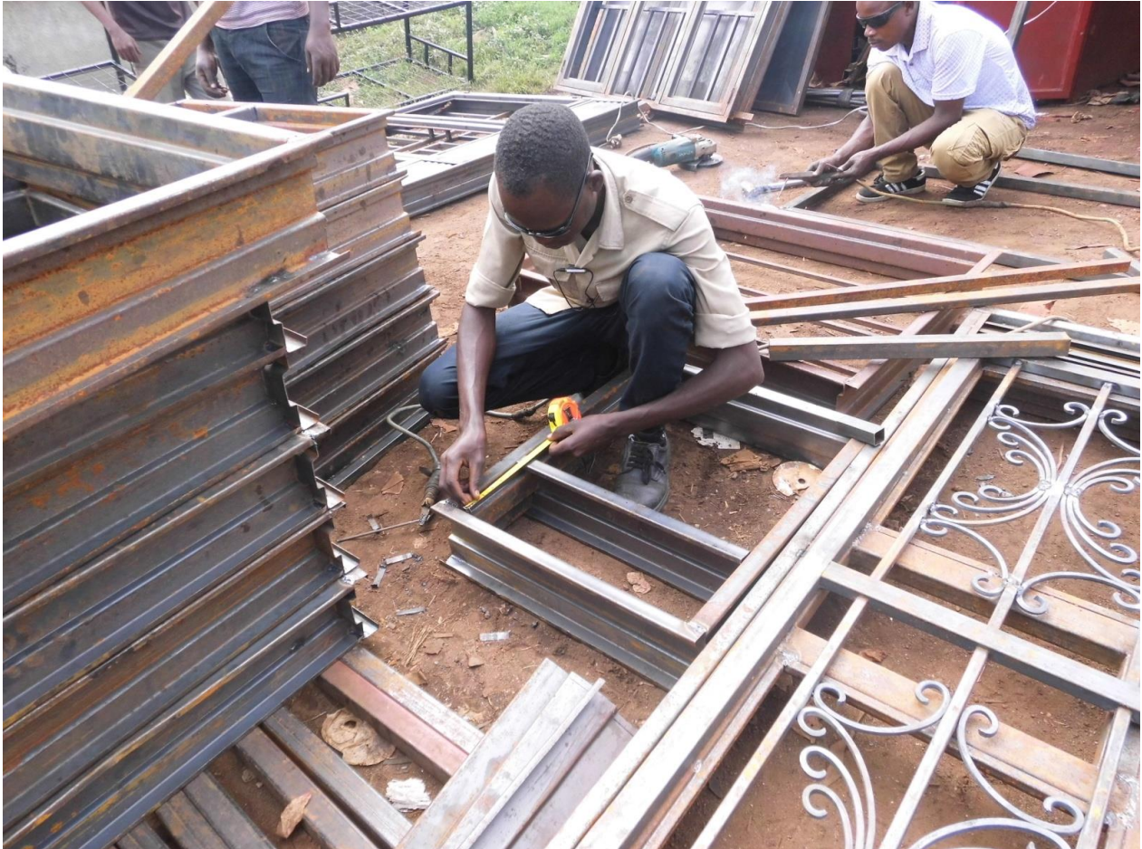
A vocational trainee in welding training workshop
